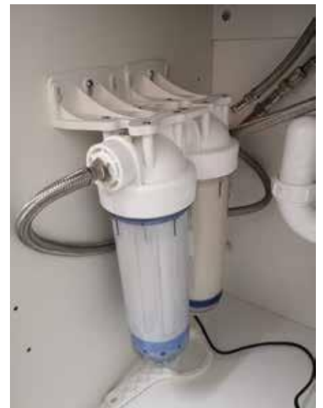
FIG1: OSMIO EZFITPRO-300 INSTALLED WITH HOSES. IT IS AN EASY WAY TO DO IT IN SOME CASES AND YOU CAN BUY THE HOSES FROM ANY PLUMBERS MERCHANT
