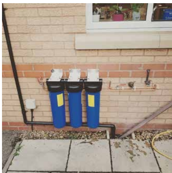
FIG 3: An example external installation before weatherproofing
